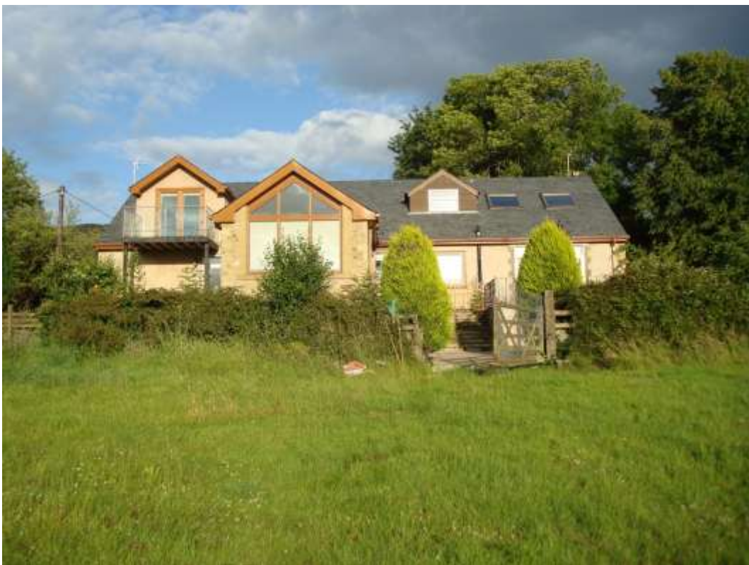
Photograph 2 – View of existing house from the north west.
