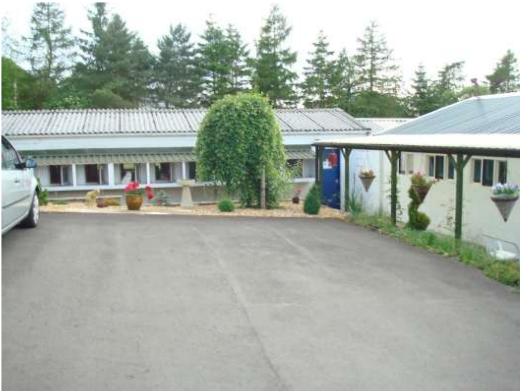
Photograph 6 – View from driveway looking south west towards kennels.
