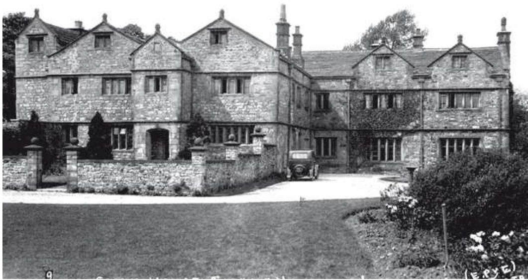
Photo E – Stirk House, Gisburn
