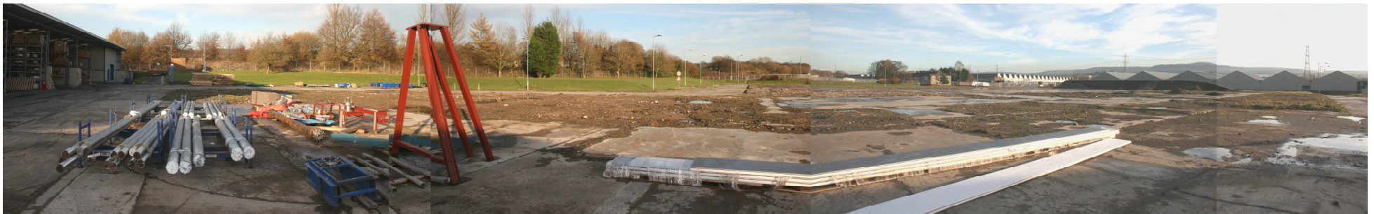
Panoramic view of the proposed application site looking south east
