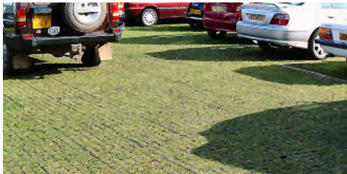
Finished Appearance of Grass Paviors
