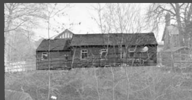
Single storey forms along Wiswell Lane.
