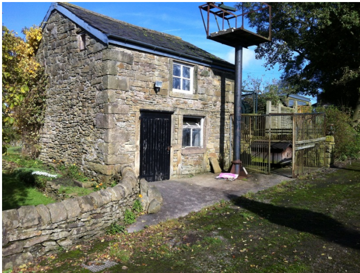
Figure 1 Outbuilding to be demolished
