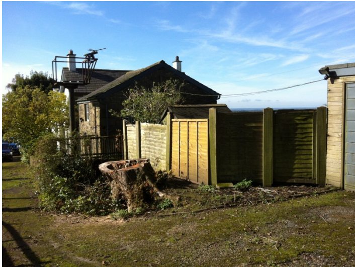
Figure 3 View of site looking West - timber garage to be demolished on right and outbuilding to be demolished in front of house
