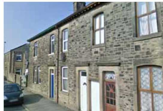
Existing development of Crumpax Avenue
