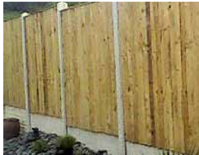
Example of fencing
