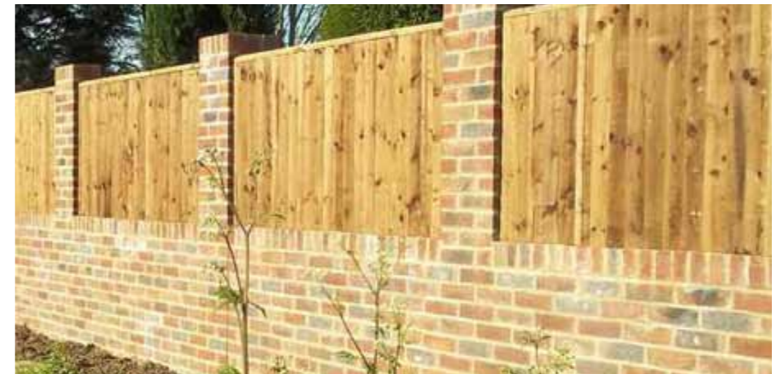
Example of brick wall with timber fence panels
