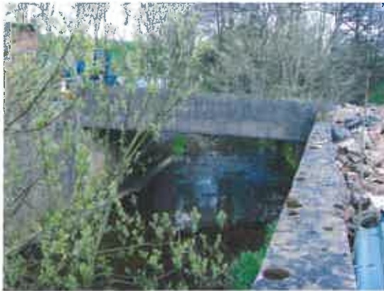
(vii) Site Bridge (3) – upstream face ISIS Unit: USBPR Flat Soffit Bridge
