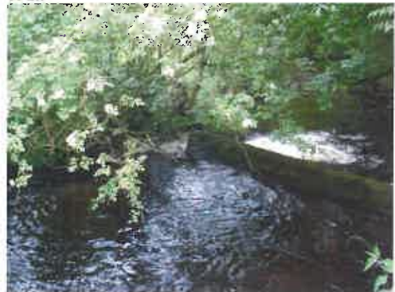
(x) Downstream weir opposite Talbot Hotel ISIS Unit: Spill unit (used to represent the third downstream, partially demolished weir)
