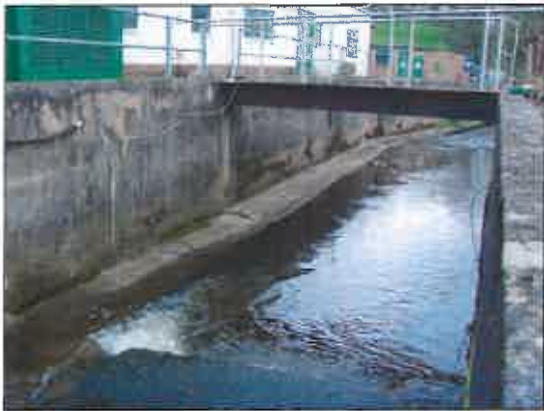
Site Bridge (2) – upstream face
