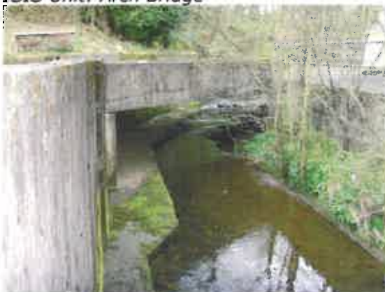
(v) Site Bridge (1) – downstream face ISIS Unit: USBPR Flat Soffit Bridge
