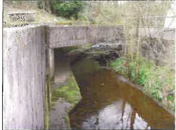
Site Bridge (1) – downstream face
