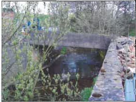
Site Bridge (3) – upstream face
