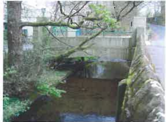
(iv) Main Access Bridge – upstream face ISIS Unit: Arch Bridge
