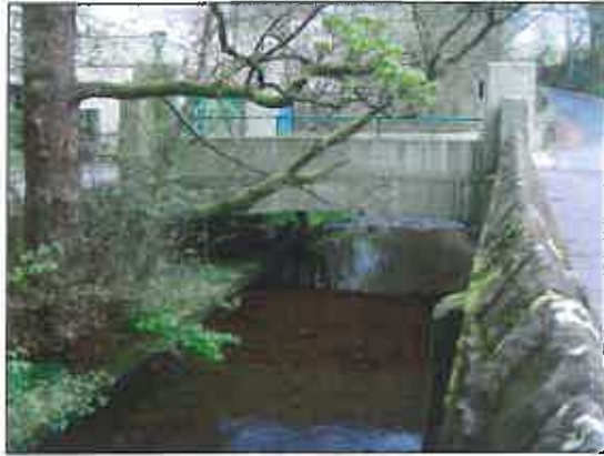
Main Access Bridge – upstream face
