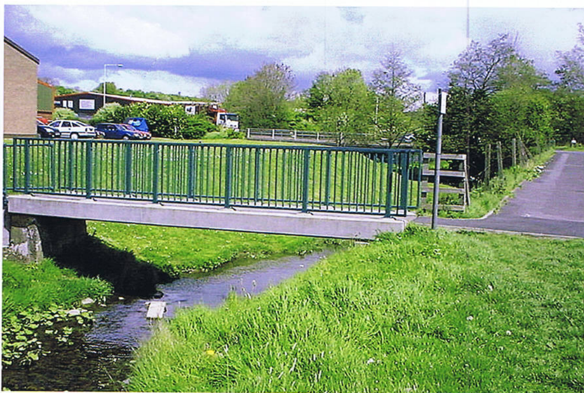
Footbridge from downstream
