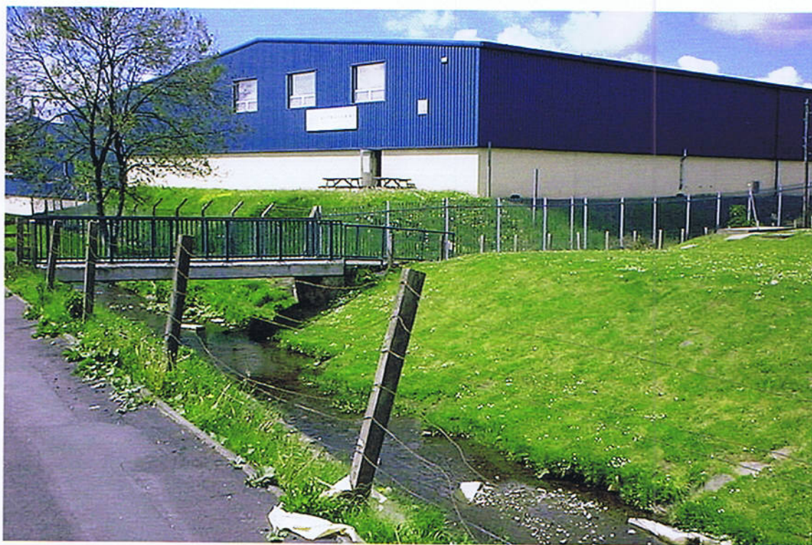
Footbridge from upstream
