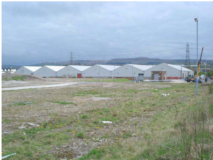
Proposed development area viewed South to existing buildings
