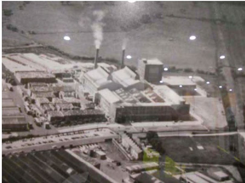
Existing Site prior to demolition
