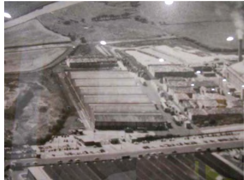
Existing Site prior to demolition
