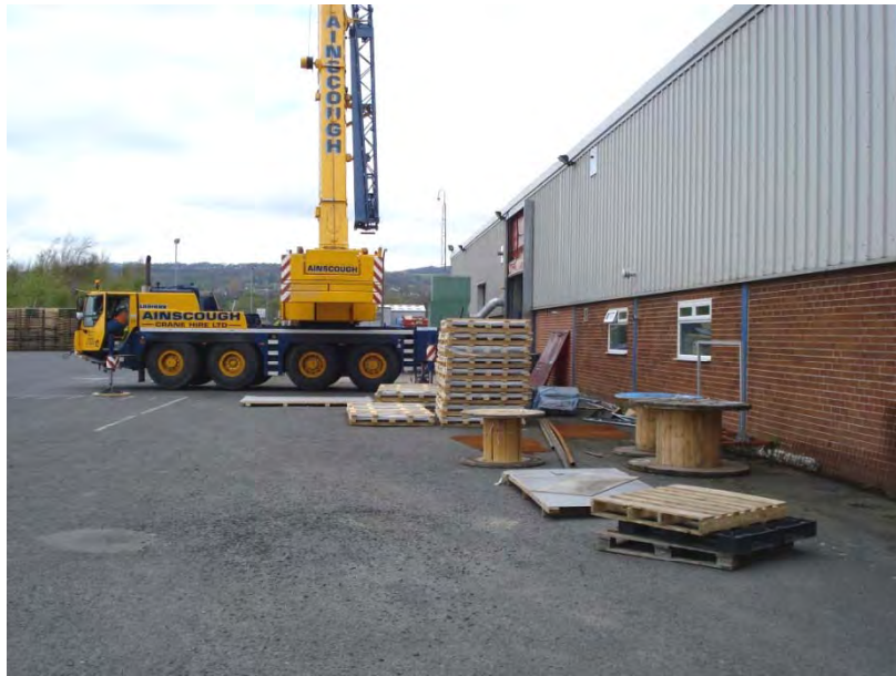
Area for Proposed Extension to existing building
