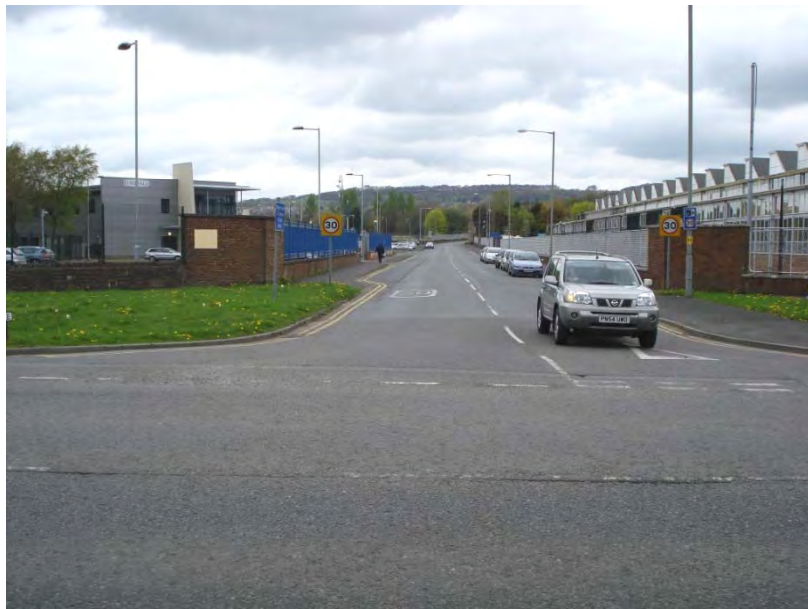
Simonstone Lane/Burnley Road junction viewed to South junction
