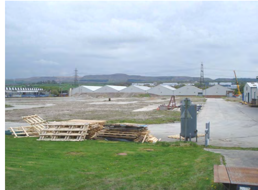
View South to existing buildings
