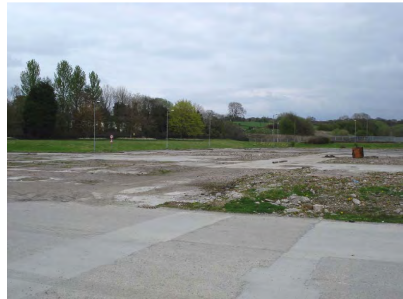
Existing Slabs and Roads on development area
