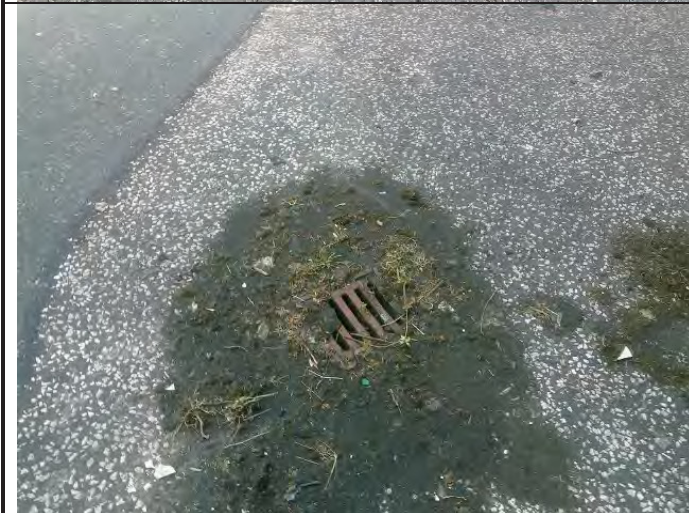
Photograph 15: Services noted on Area 1.
