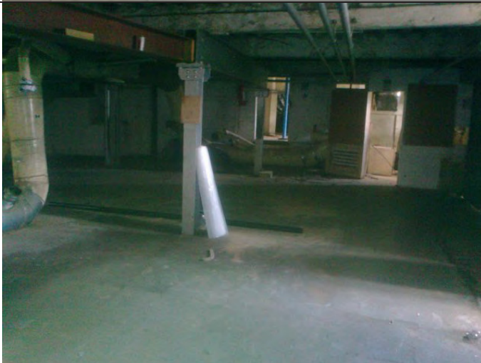
Photograph 3: Inside mill building showing thick concrete floors.
