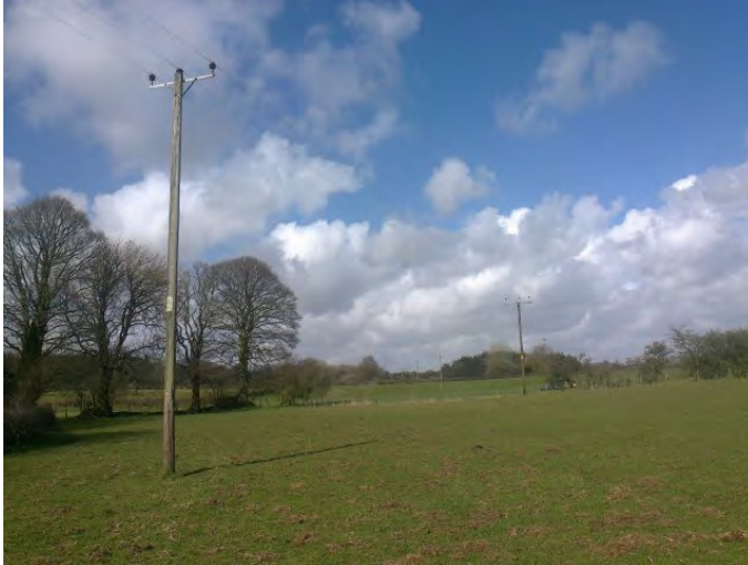
Photograph 25 (facing N): Electricity pylon running though Area 4.
