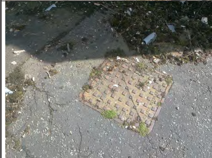
Photograph 14: Services noted on Area 1.
