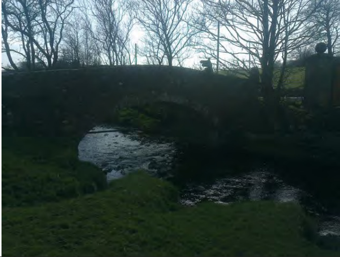
Photograph 22 (facing S): Footbridge from Longridge Road onto Area 4.
