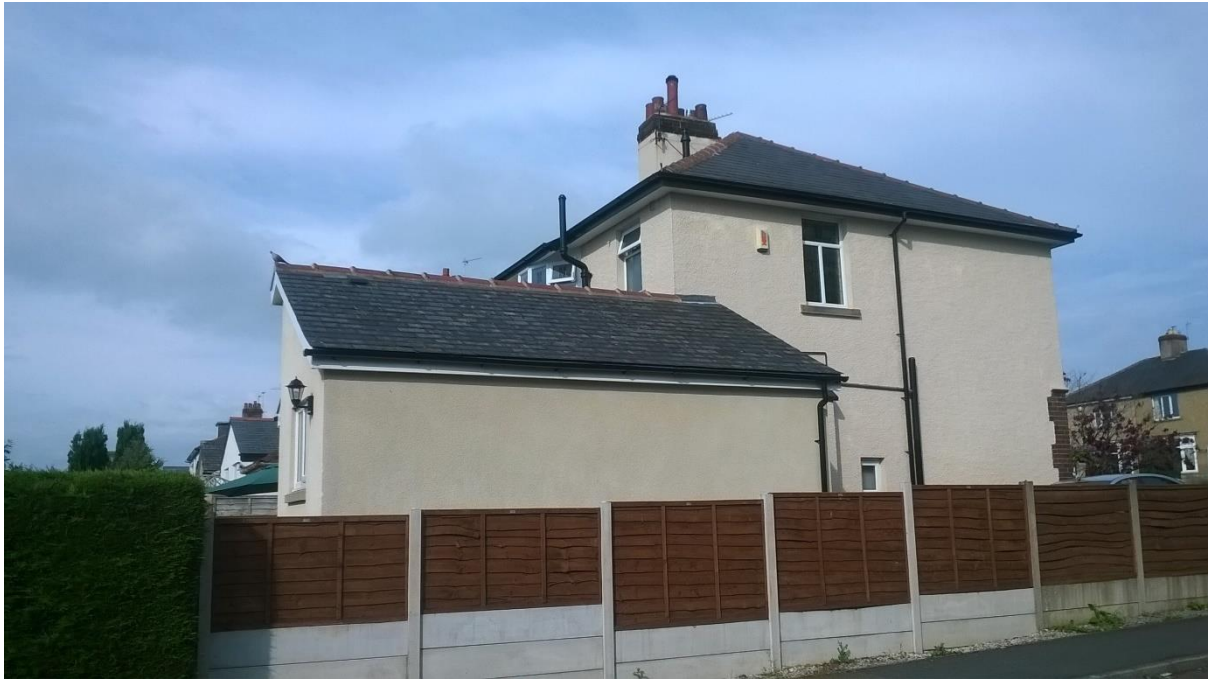
F. Plain render on new and old has enabled the new building here to blend with the existing, rather than new and old be kept separate or the new build forced to adopt the original style and design; in this case it would have been to repeat a pebble-dash. This example is 99 Chatburn Road.
