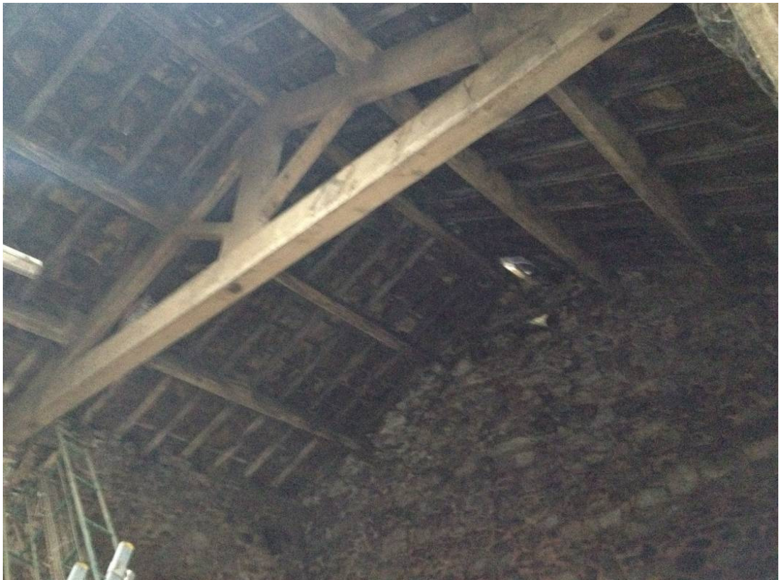
Figure 6: Barn Roof and Timber Beams
