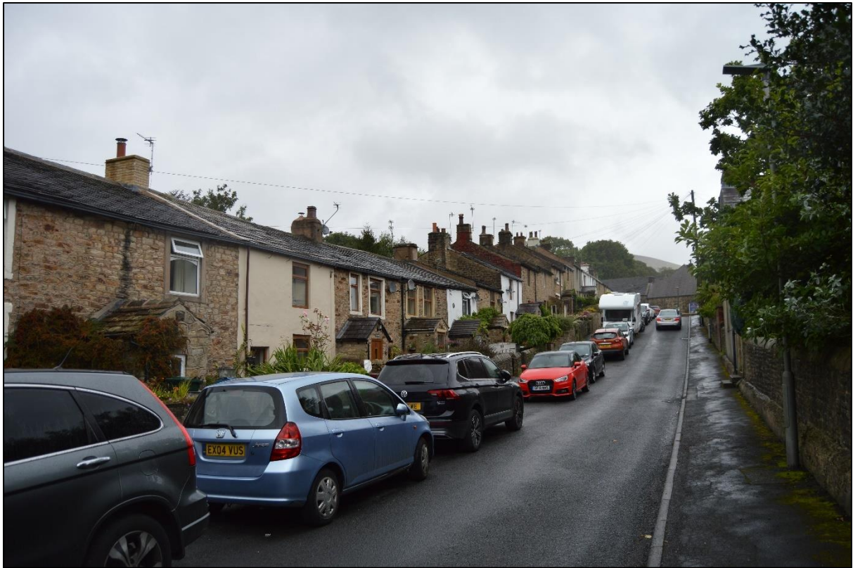
PL15: View of cottages on the north side of Wesley Street.
