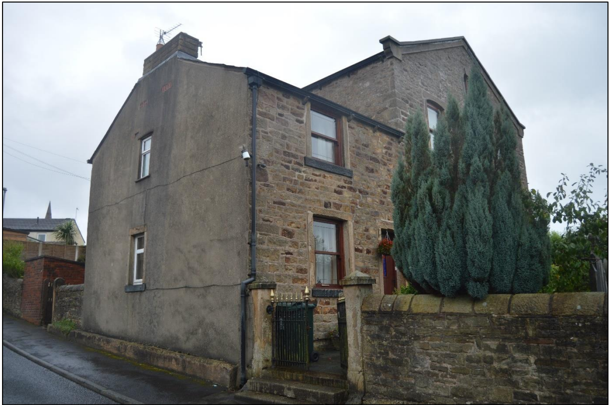
PL09: View of the north west facing elevation of the now converted former Sunday school.
