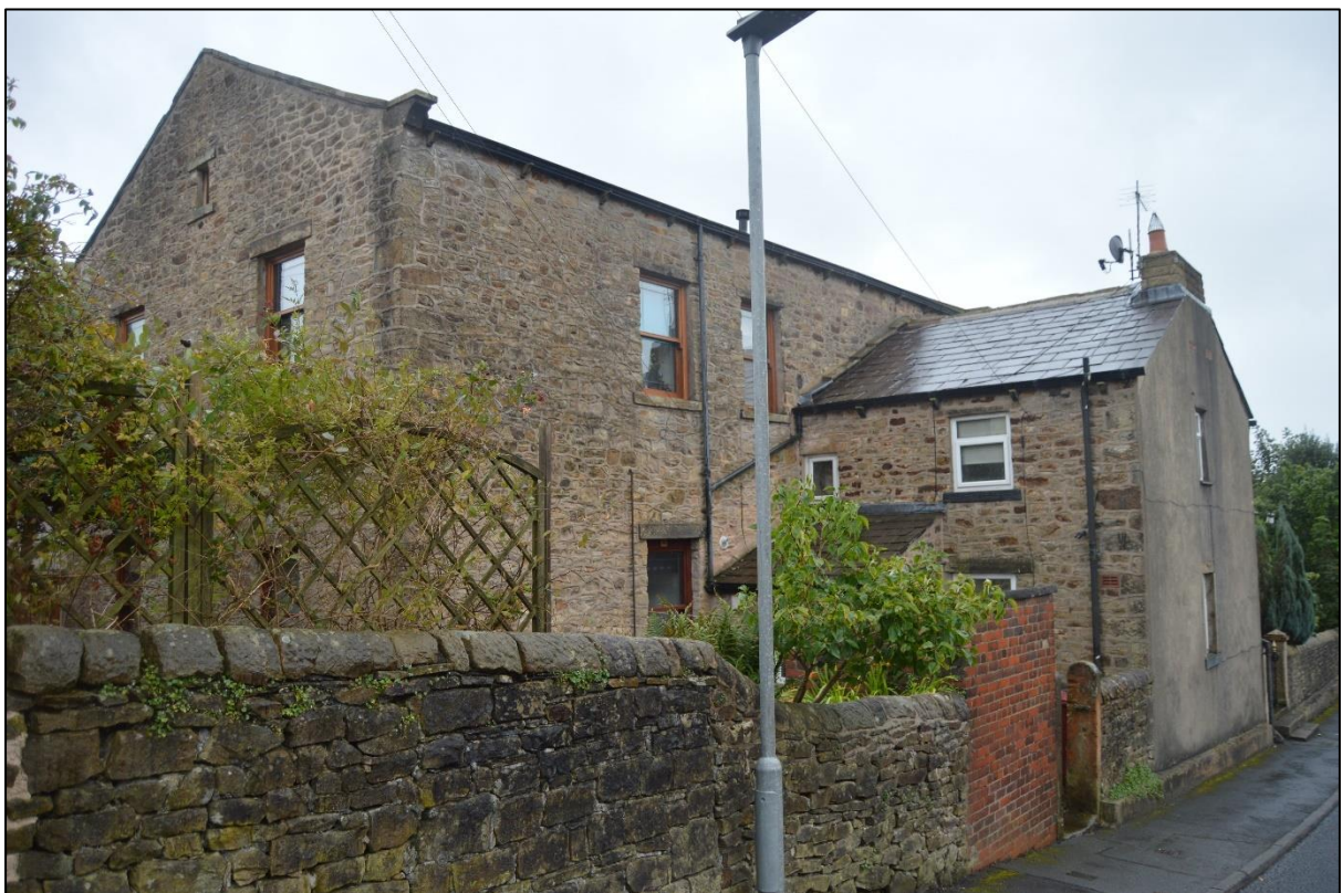
PL10: View of the north east facing elevation of the now converted former Sunday school.
