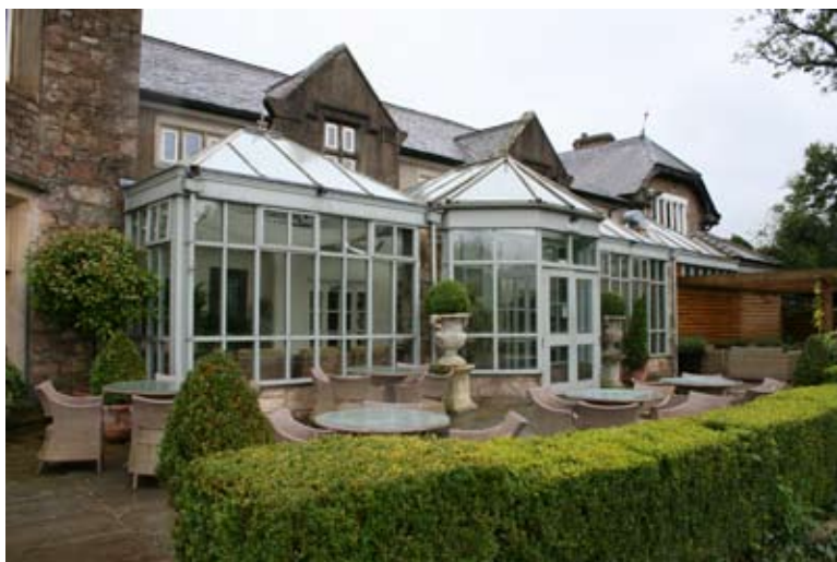
Photograph 4. The present conservatory at the rear of the function room block.
