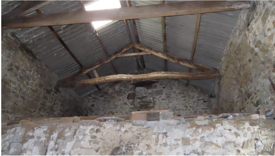
12. Closed hay forking door evident in the former gable of the barn, now forming the left (west) wall of the trap house
