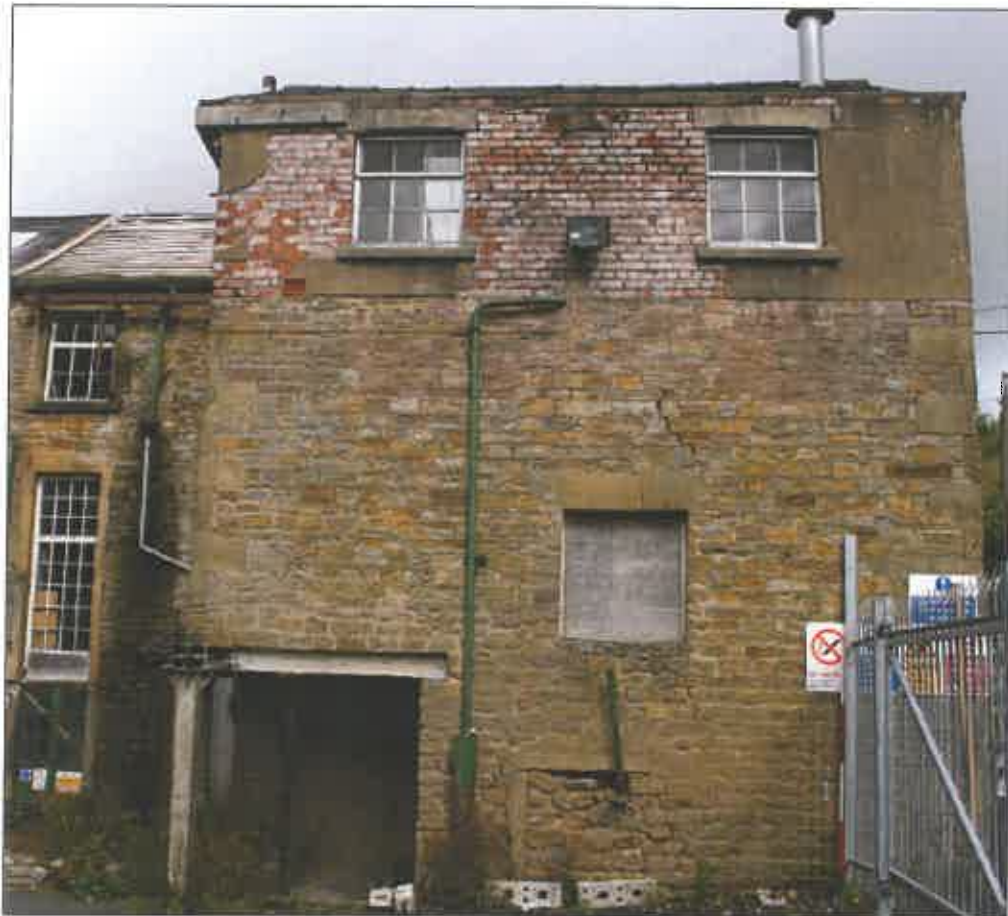
Plate 15: The remodelled southern extension to the main mill block
