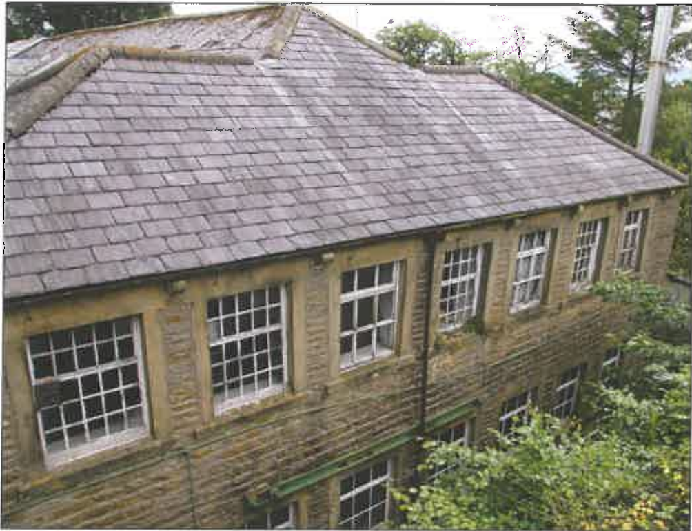
Plate 10: External west elevation of the west wing
