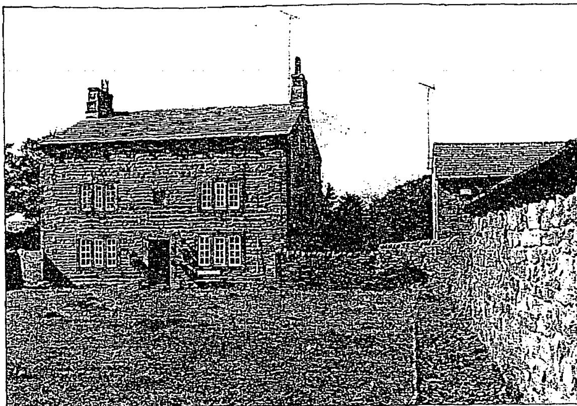
Photo 3: Front elevation of the house, from the east
