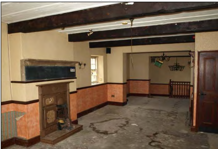
Photo 12: Ground floor of east wing (G6), with early 19th century plank and muntin ceiling and kitchen fireplace, and mid 20th century range
