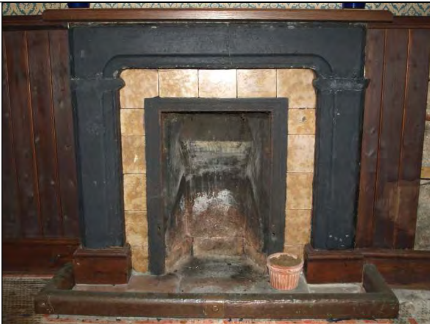
Photo 11: Fireplace in bar (room G2): original stone surround with later infill and fender
