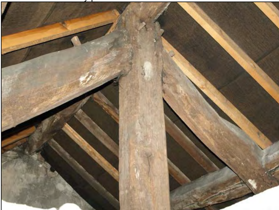
Photo 23: King post of pegged roof truss in 1779 building
