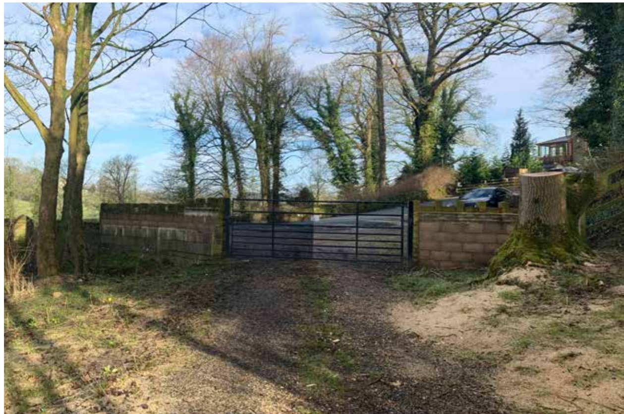
Existing site entrance from the highway. Entrance walls not in client ownership. Material selection not of client.
