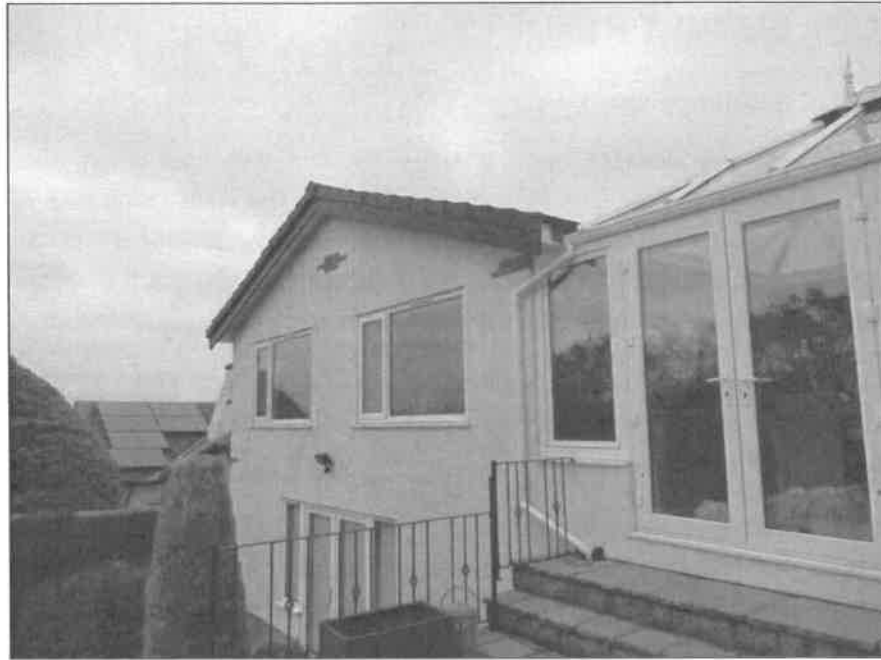
Plate 2: The rear of the building comprised of a conservatory and white stucco plaster.
