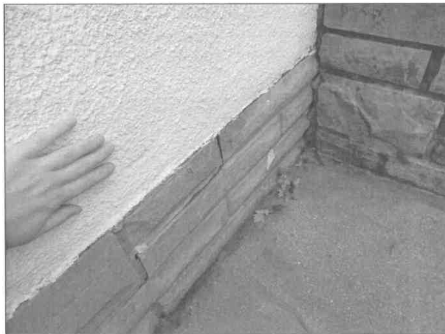
Plate 3: The white stucco walls would have been an ideal surface for bat droppings to adhere to, however despite a thorough inspection no evidence was found.
