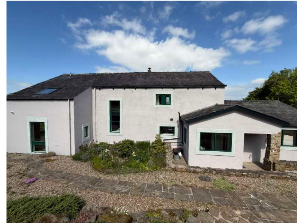
South-East elevation and rear entrance porch.
