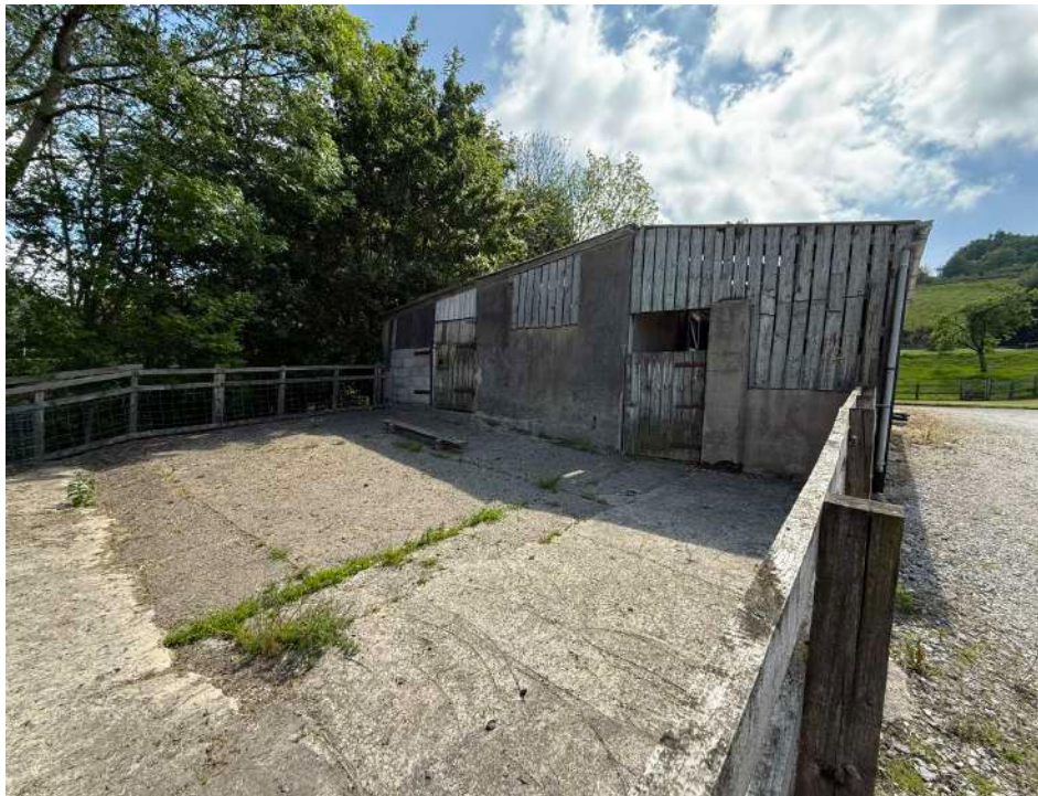
Outbuilding and stable yard.
