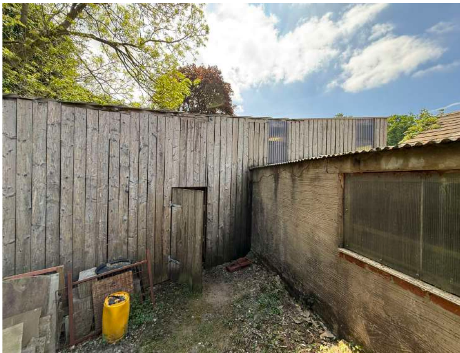
Rear of outbuilding.
