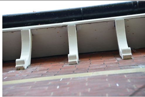
Photo 5.5 A view beneath the eaves showing gaps between the wooden soffits and brickwork where bats could feasibly enter
