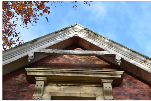
Photo 5.3 Detailed view of the bargeboards and soffits on the south-facing gable end
