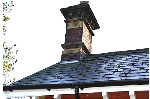
Photo 5.6 Detailed view of the raised ridge tiles and slates on the single storey section of the building and raised lead flashing at the base of the chimneystack
