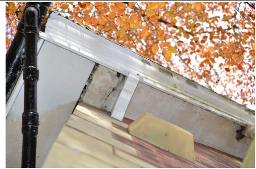
Photo 5.4 View beneath the eaves showing potential access points for bats in the soffits
