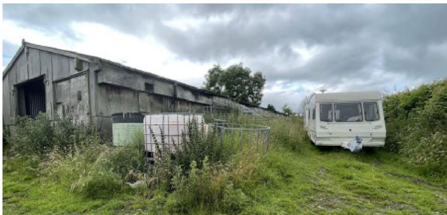
Photograph 2 above: Existing storage / garage building on site
