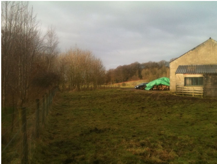
Recently planted tree belt (to left) screening the gravel works building from public highway
