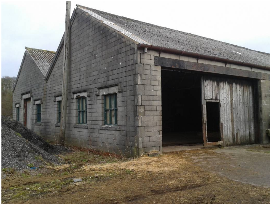
Present substantial (concrete walled) construction. The replacement scheme proposes natural stone walls
