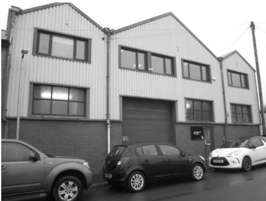
2 Elevation to Warwick Street
