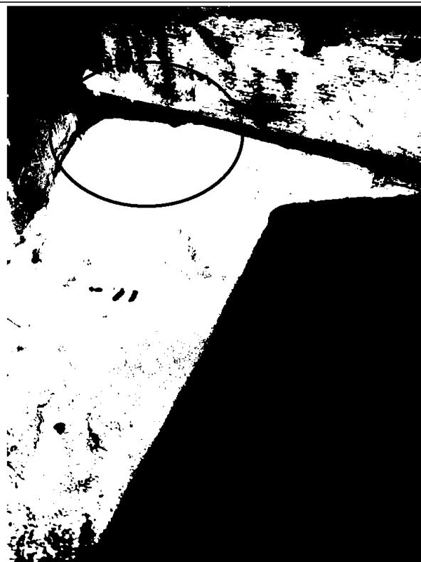
Photo 15: Gap at the top of the dividing wall above the bat droppings
