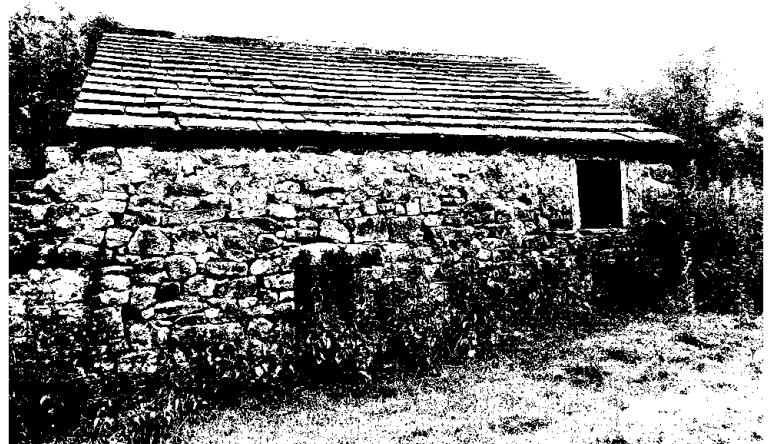
The store has well sealed walls and a stone slate roof. It is a small building which could be fully inspected during the daytime surveys
