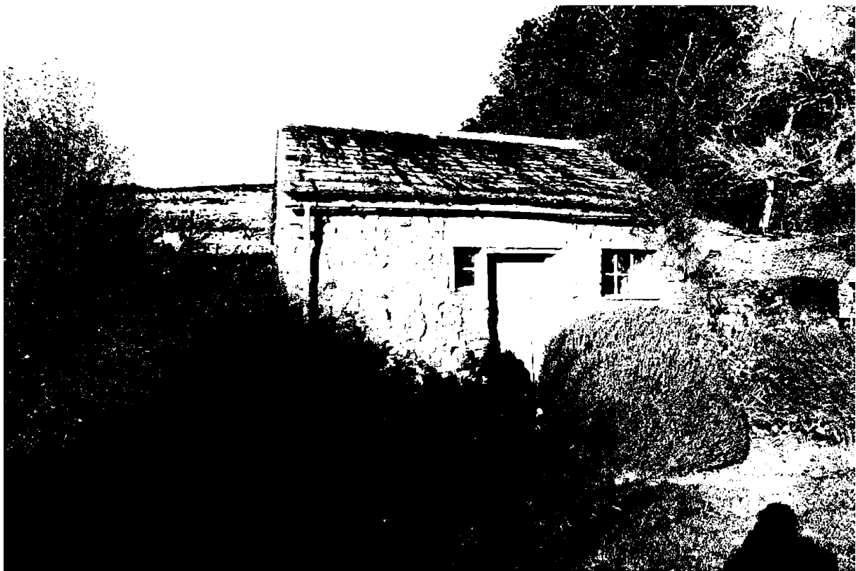
Plate 25: Outbuilding, facing north-west
