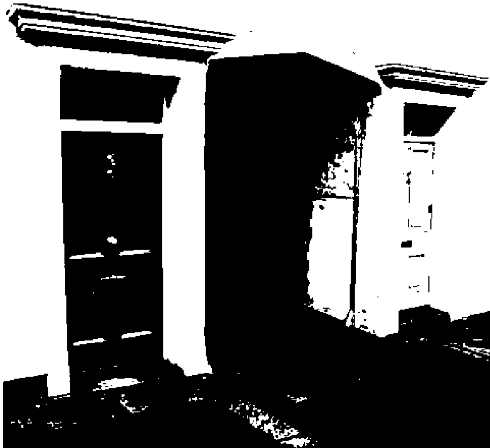
Pl.3: The front entrance to the cartway – note pintle hooks on both jambs.
