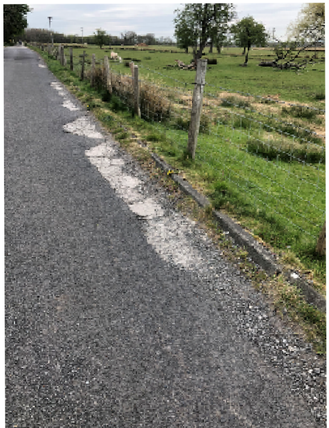
Road damage which is collapsing into the farmers field which has a poorly maintained fence.
