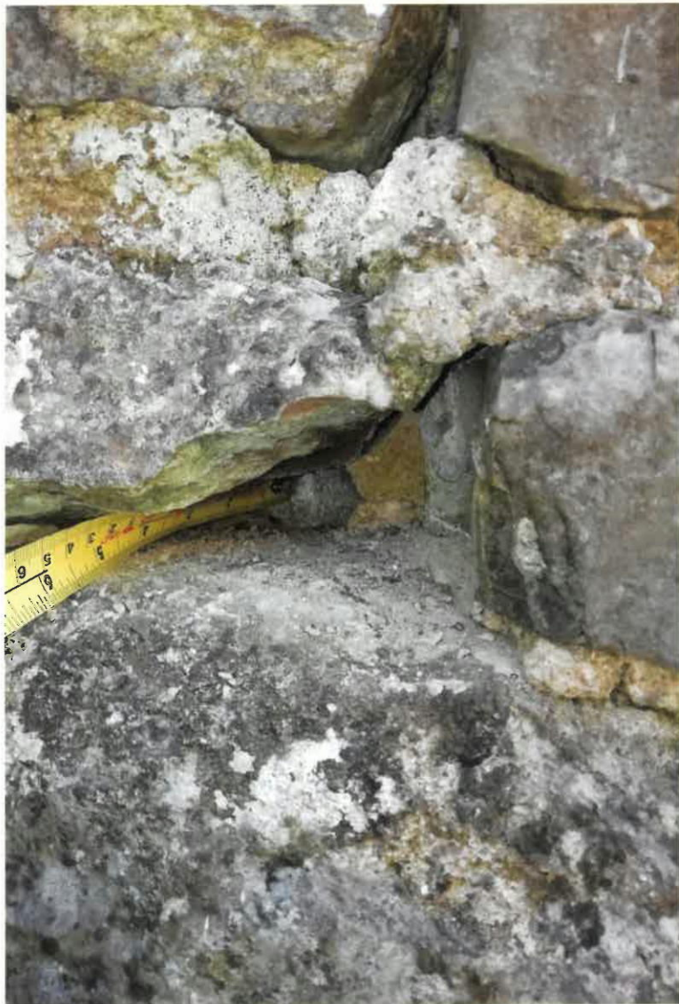
Tape measure abutting cement blockwork inner wall of modern outbuilding, confirming façade 15cm deep
