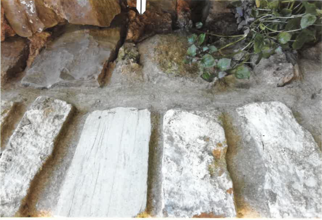
Former coal shed wall of 6 Downham Rd just visible
