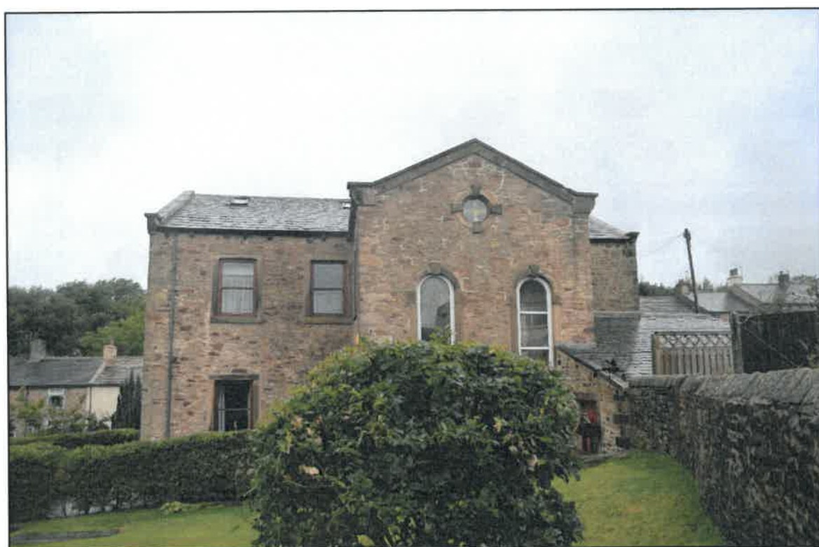
PL08: View of the south east facing elevation of the now converted former Sunday school.
