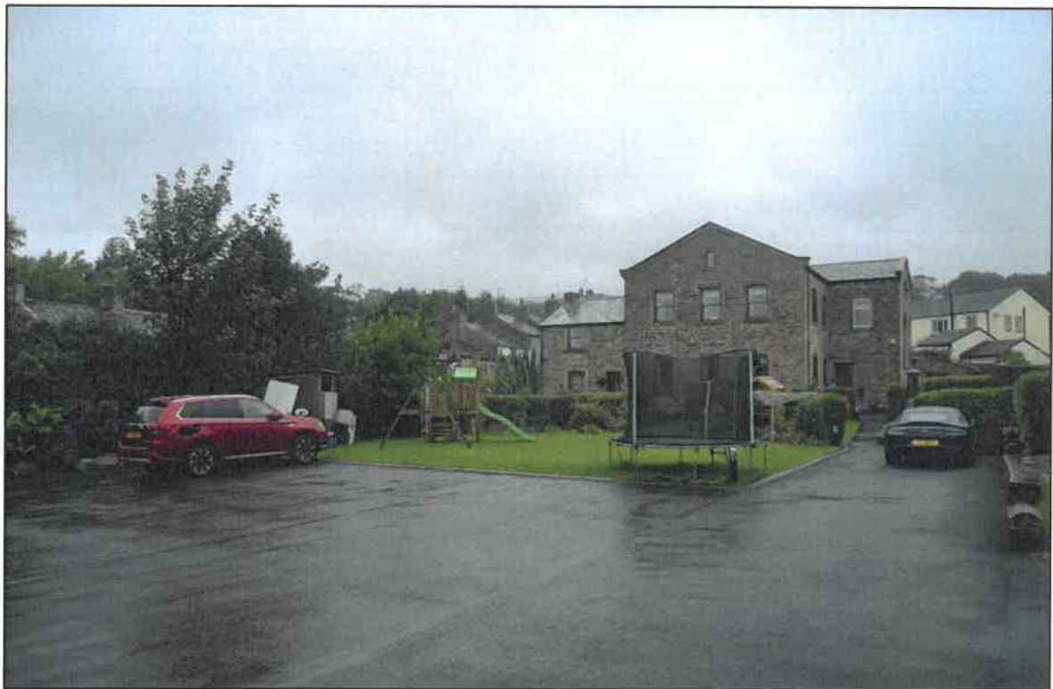
PL03: View north east within the site.
