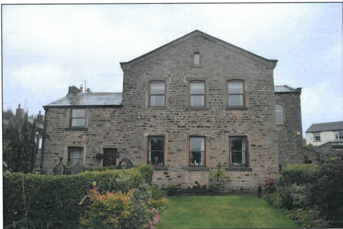
PL07: View of the south west facing elevation of the now converted former Sunday school.
