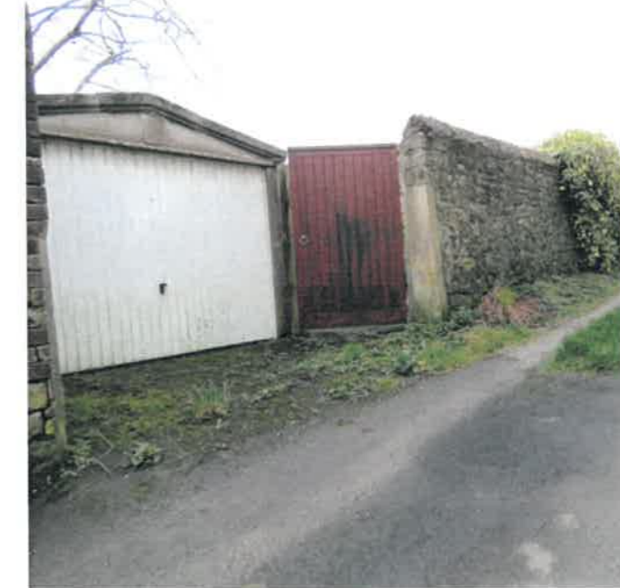
Access off service lane.
