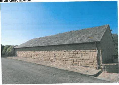
The garage is a stone built modern single story building with a double pitched slate roof. General condition of the building is very good, with no missing pointing between stonework, no missing or slipped slates on the roofs, and no gaps on
