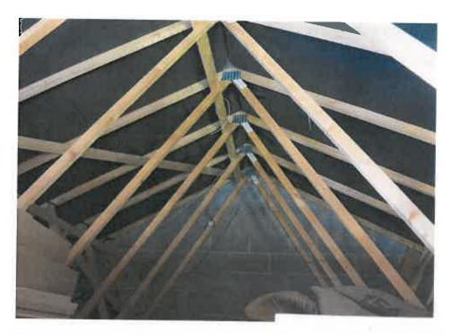
Underfelt is all in good condition with no rips or tears. The interior of the garage is well lit with no access to crevices or gaps in the block work walls.
