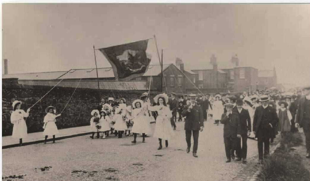
Figure 1 Church of England Parade - Mill in background with 3 windows at first floor
