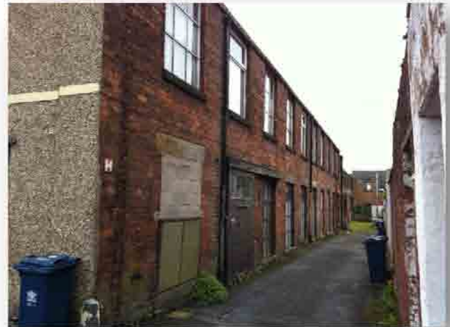
Figure 2 West Elevation down side alley
