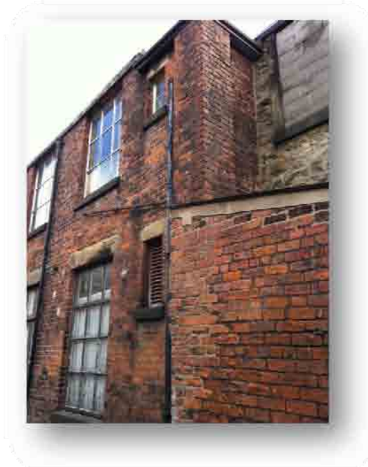
Figure 3 West Elevation down side alley
