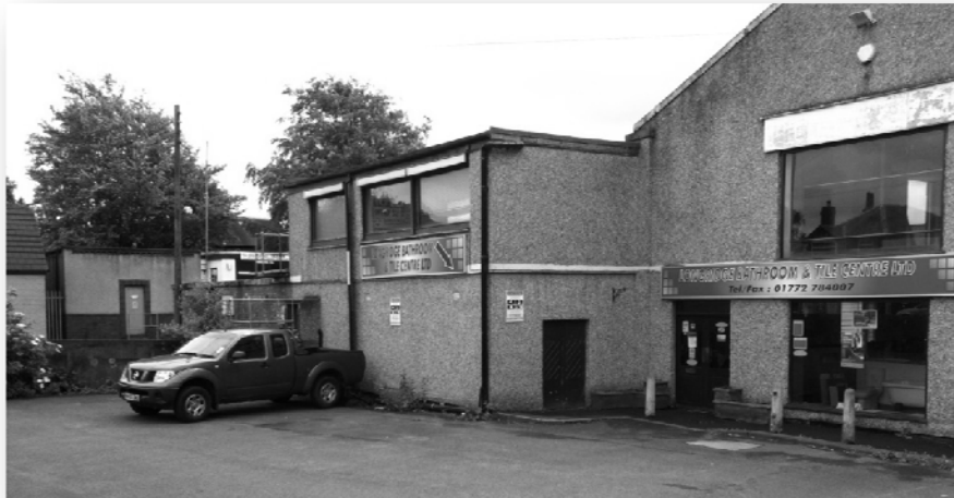
Figure 5 Heavily rendered elevations and ill-conceived signage
