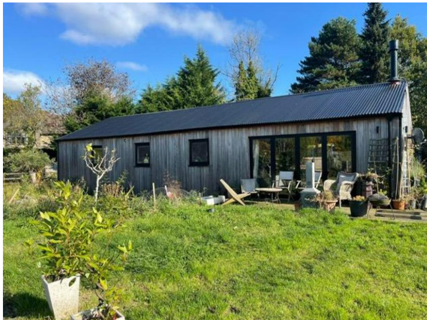
Figure 6 – Site photograph of the dwelling
