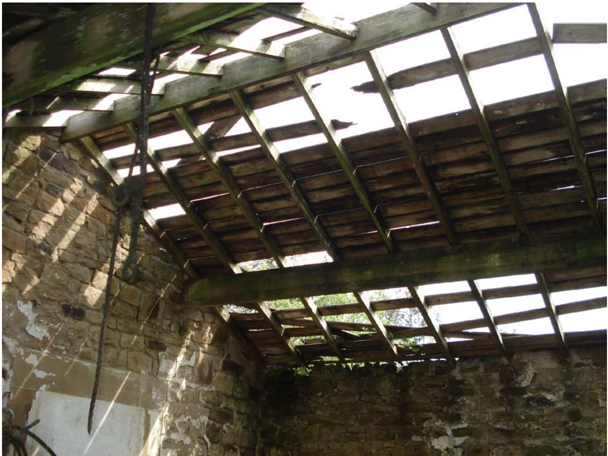
Plate 33– Store 5 roof viewed internally
