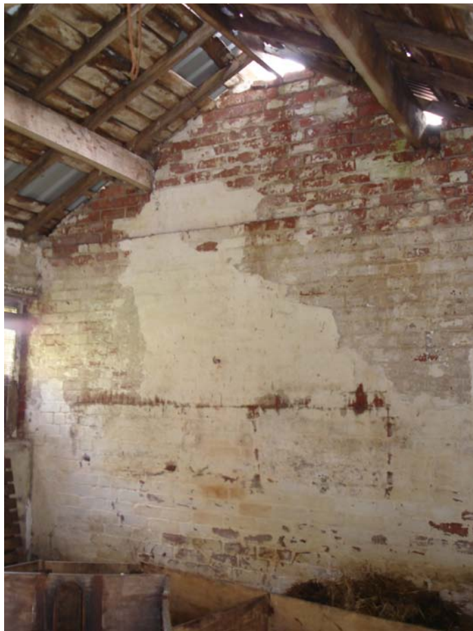
Plate 27 – Store 3 internal brickwork partition to Store 4
