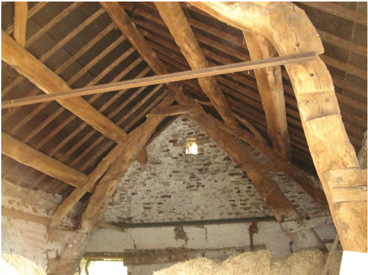
Plate 18 – Main Barn 'Cruck' frames (north facing)
