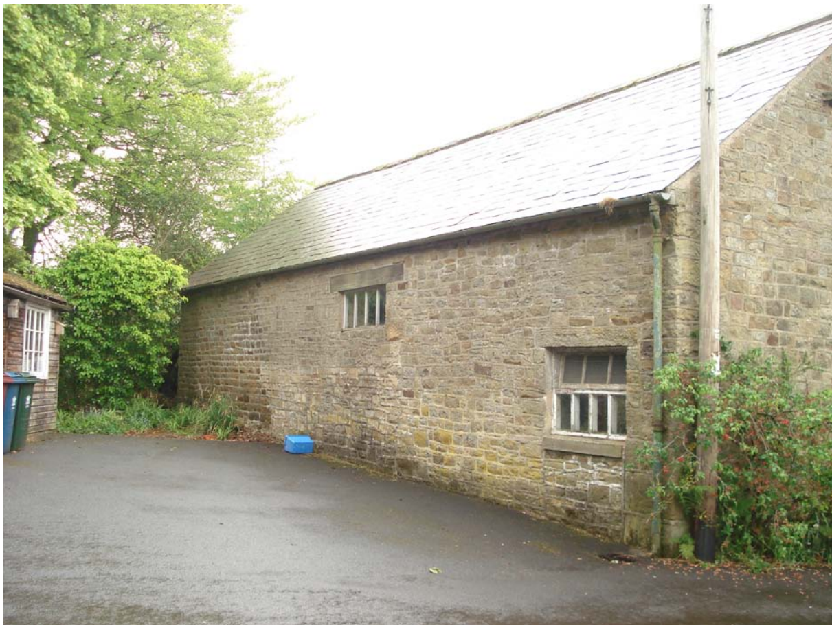
Plate 01 – Main Barn rear elevation
