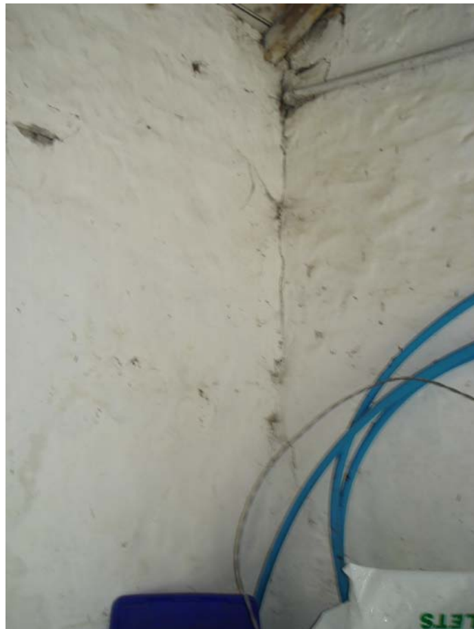
Plate 26 – Store 2/3 internal partition butt joint with rear elevation
