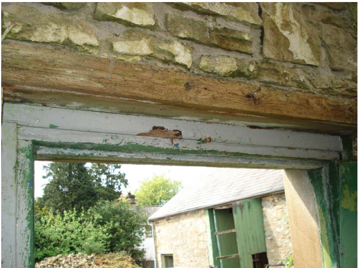
Plate 31– Store 4 timber lintel member (front elevation)
