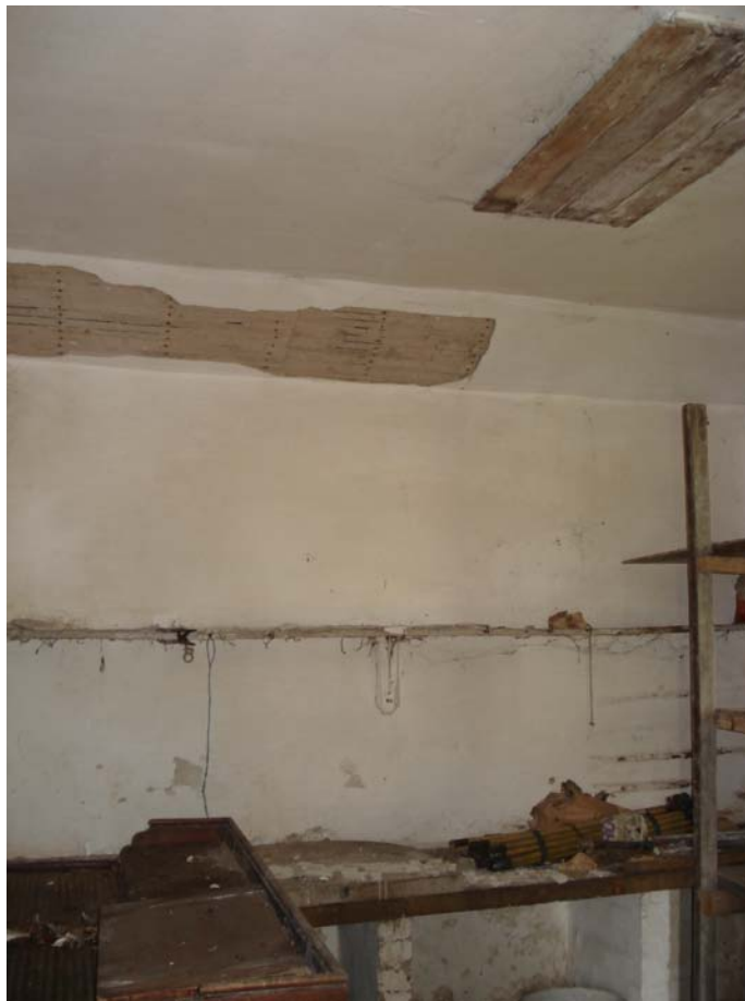
Plate 23 – Spalled ceiling finishes within Store 1
