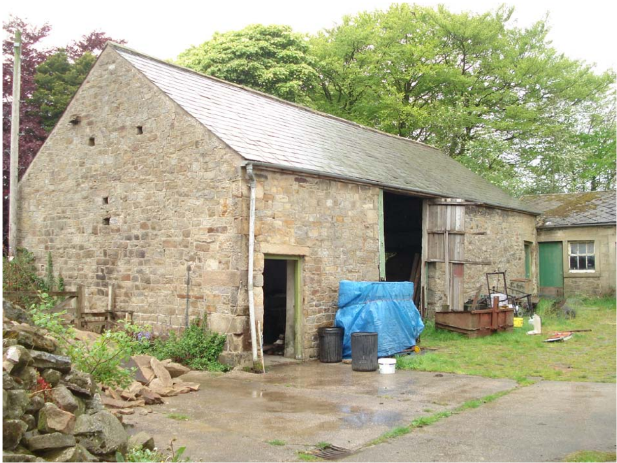
Plate 05 – Barn Gable and Front elevations
