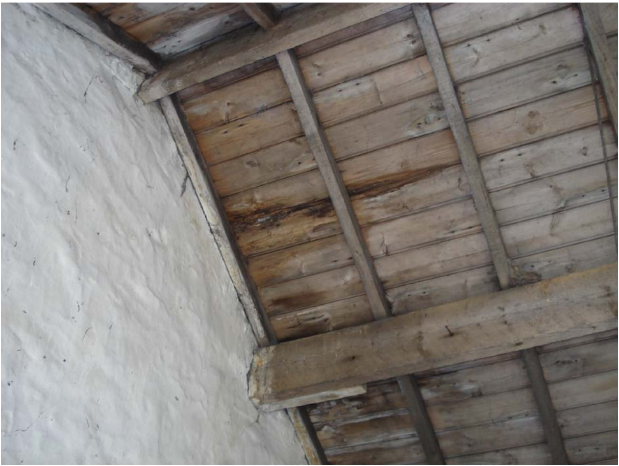
Plate 25 – Store 2 internal roof finishes
