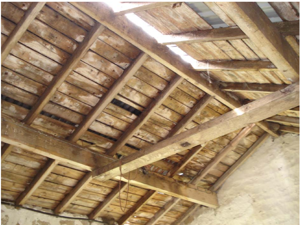
Plate 29 – Store 3 internal roof finishes
