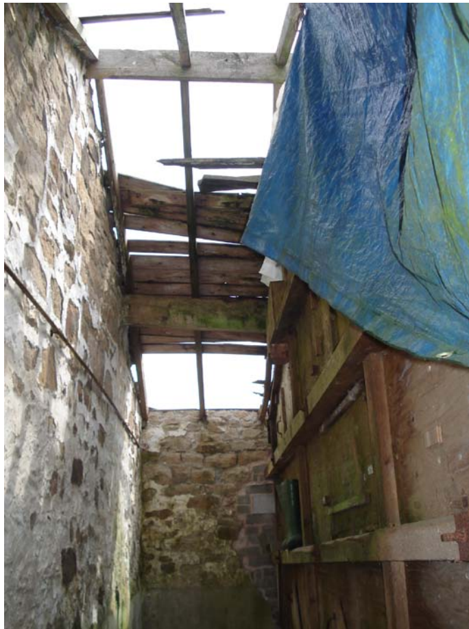
Plate 35 – Store 6 internal partition and roof adjacent to Store 5
