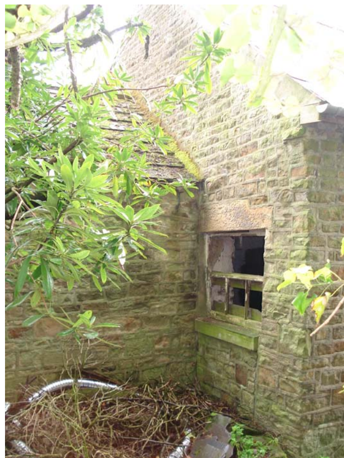
Plate 14 – Infilled former door within Barn north gable elevation
