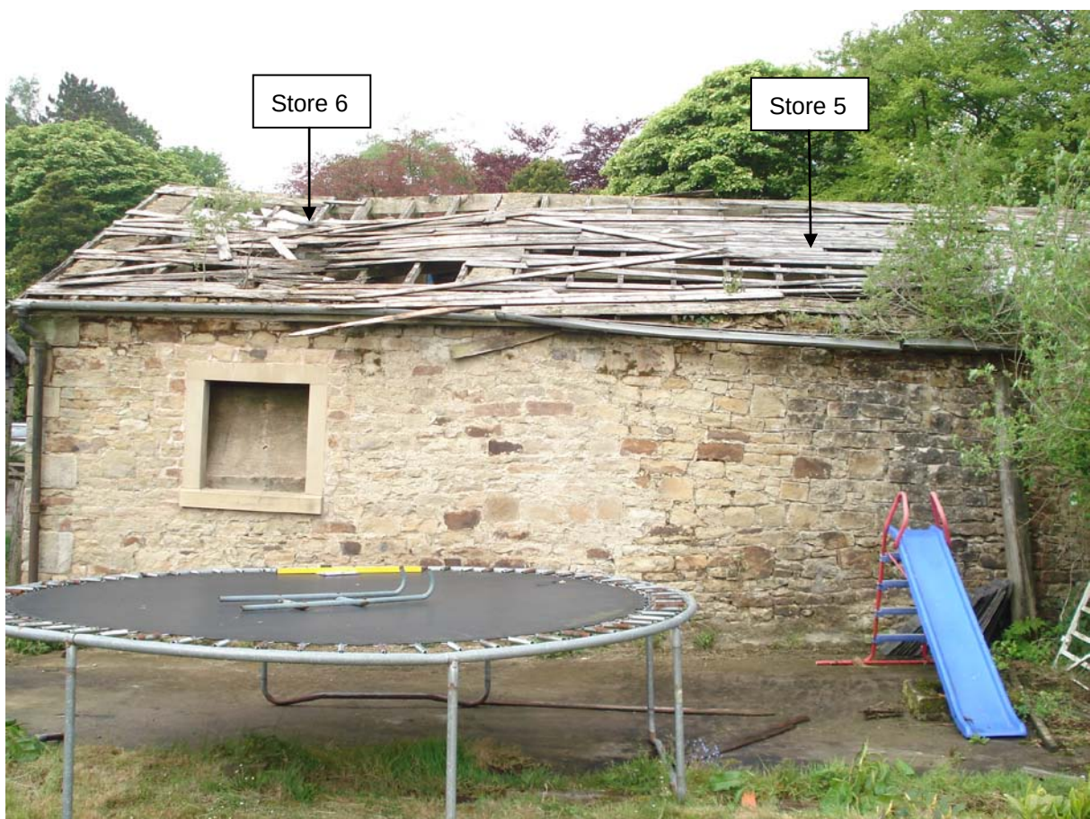
Plate 12 – Stores 5 & 6 rear elevation
