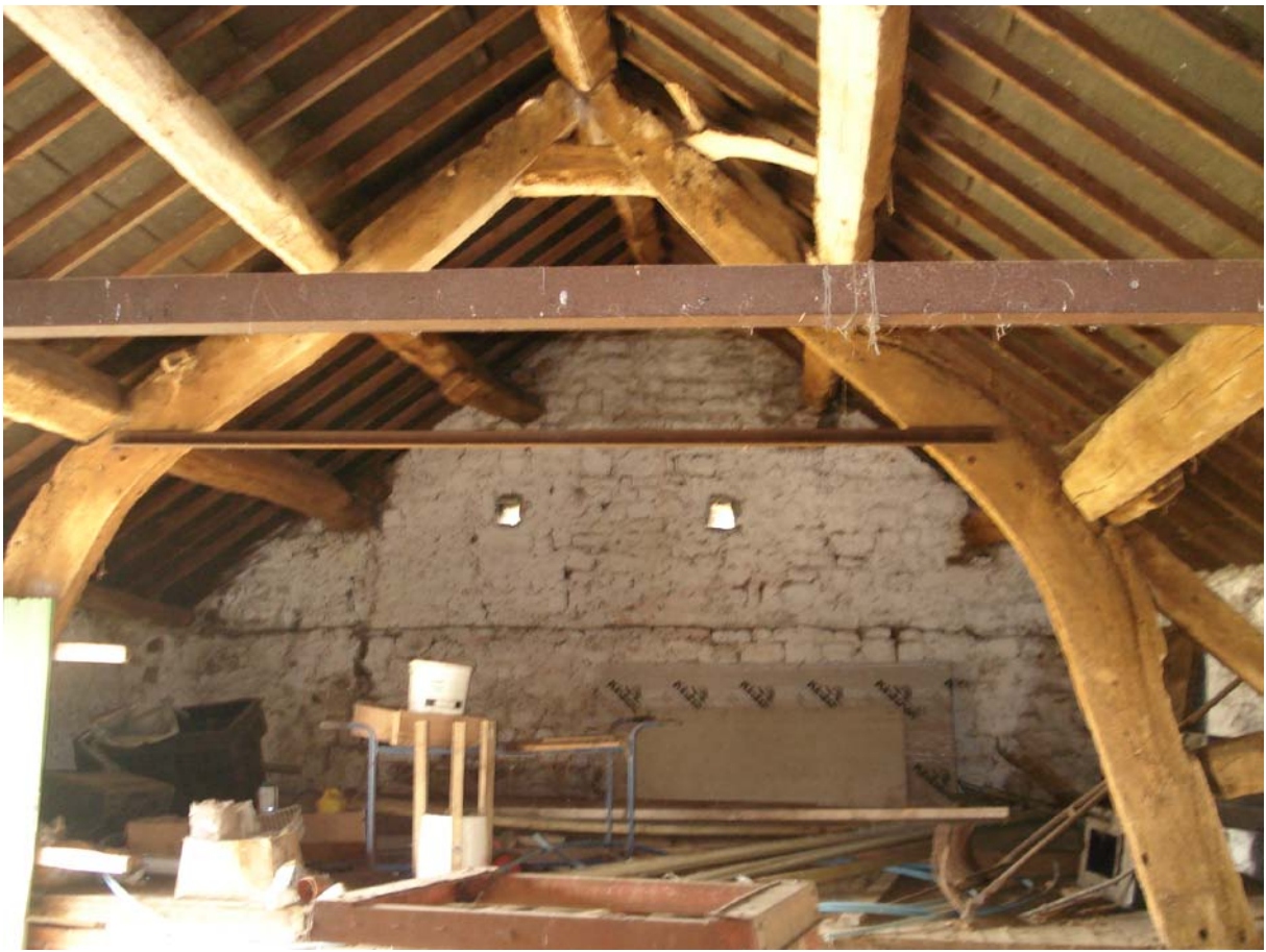
Plate 19 – Main Barn 'Cruck' frames (south facing)
