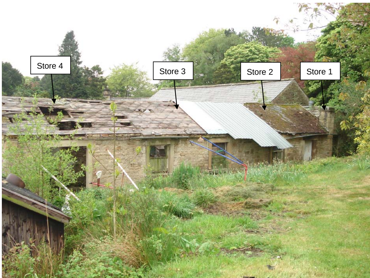
Plate 13 – Stores (northern) rear elevation
