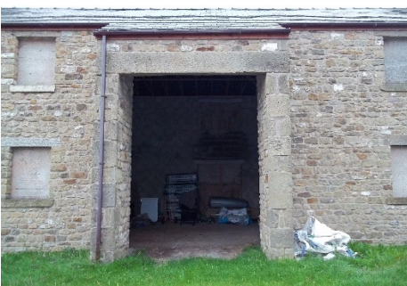
Figure 10: Building #5 (north-east gable end)
