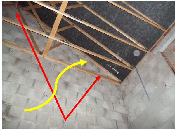
Figure 14: SW gable end
