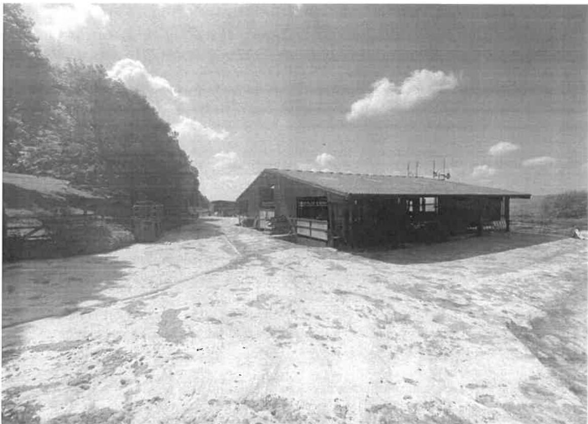
View of the site on arrival down the access track
