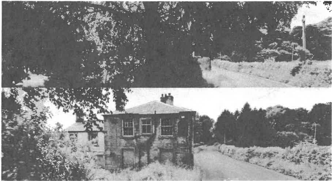
Figure 18) Views on approach from the east
