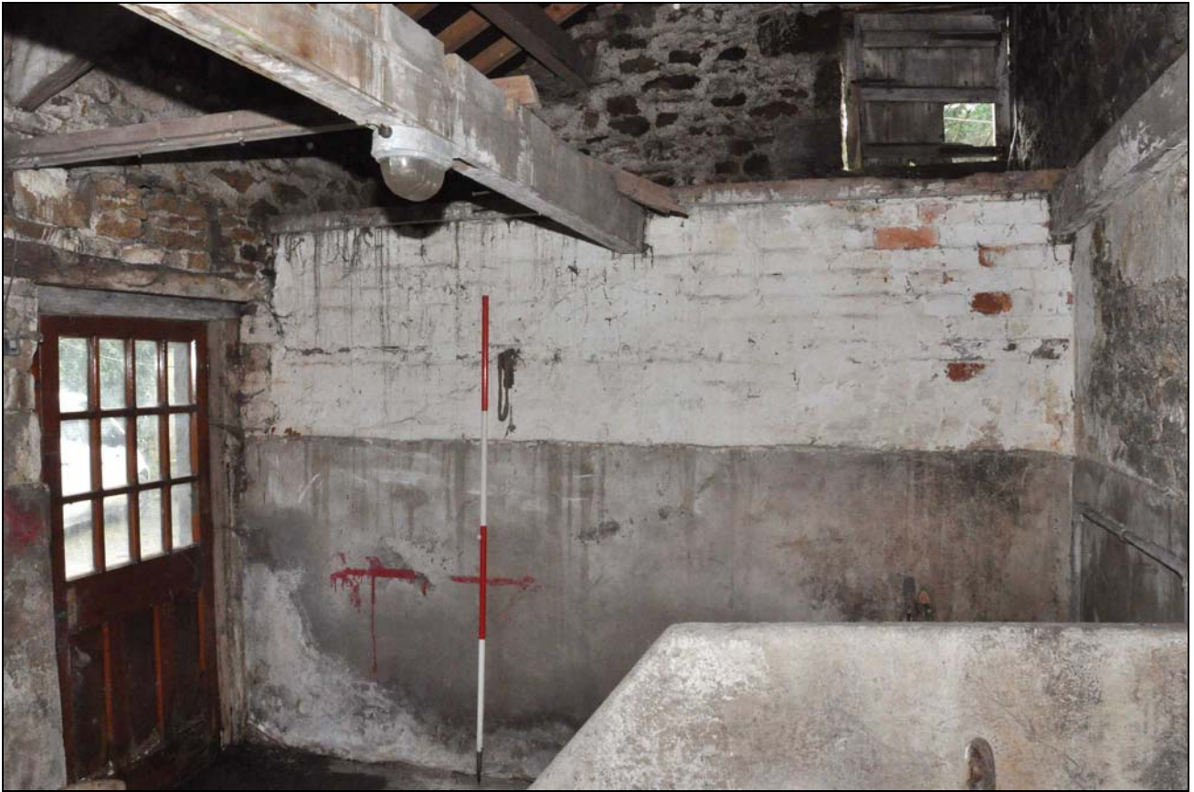
Photo 29: Former stable in outshut, from the north-west
