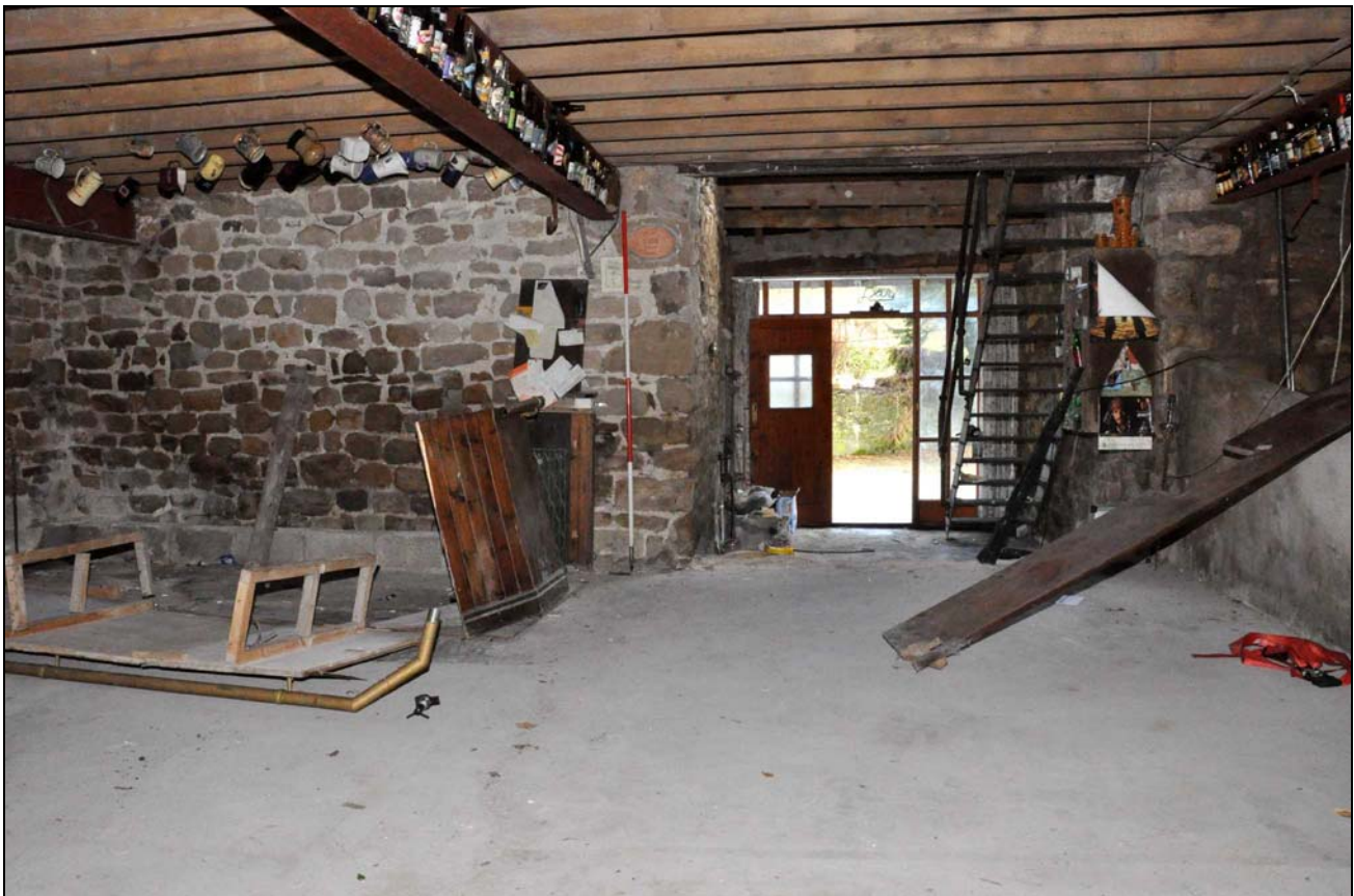
Photo 15: Interior of barn, ground floor, north-east corner with entrance from porch
