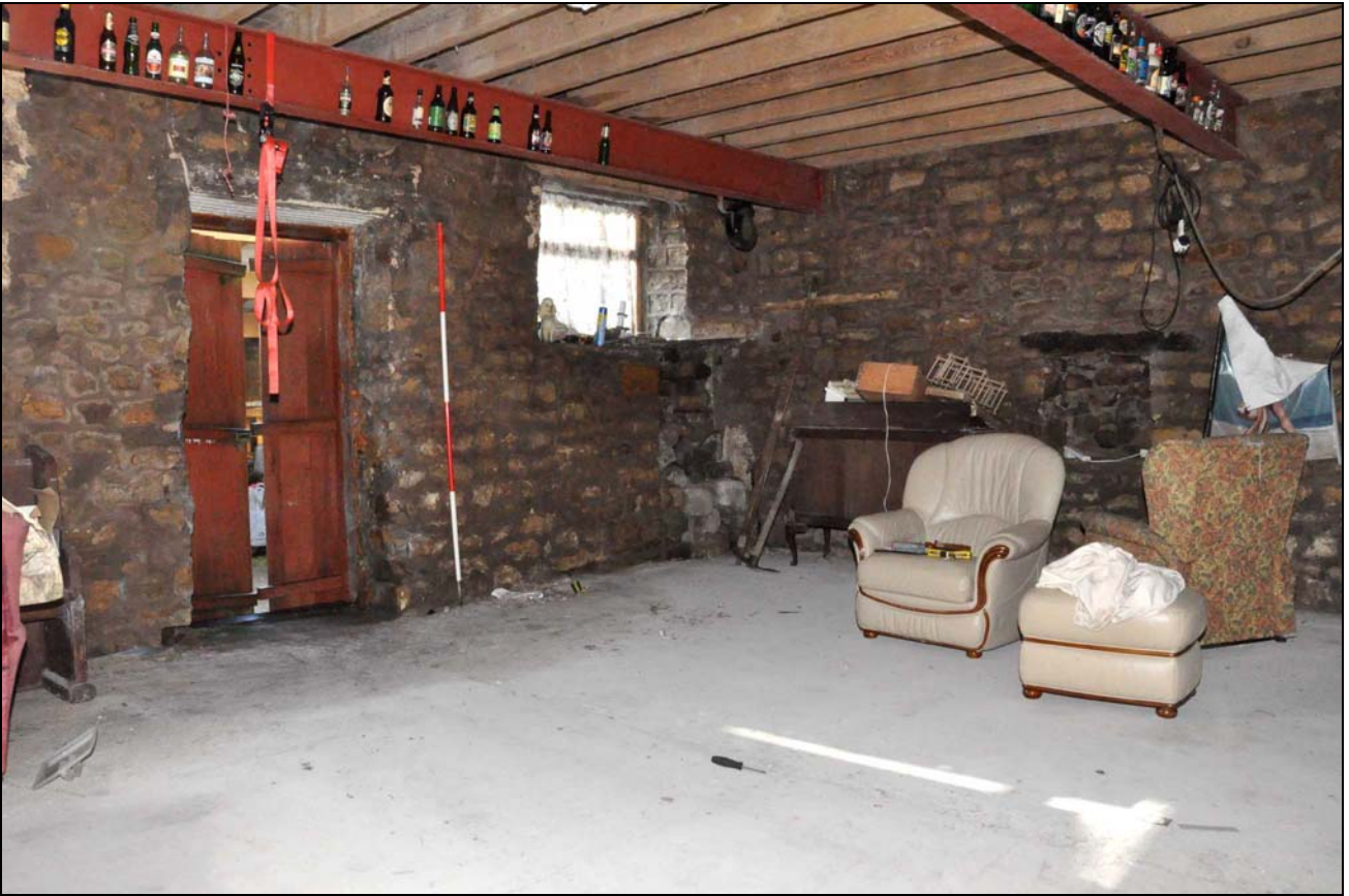
Photo 17: Interior of barn, ground floor, south-west corner
