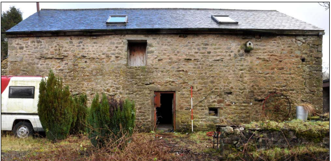
Photo 6: The barn, from the west
