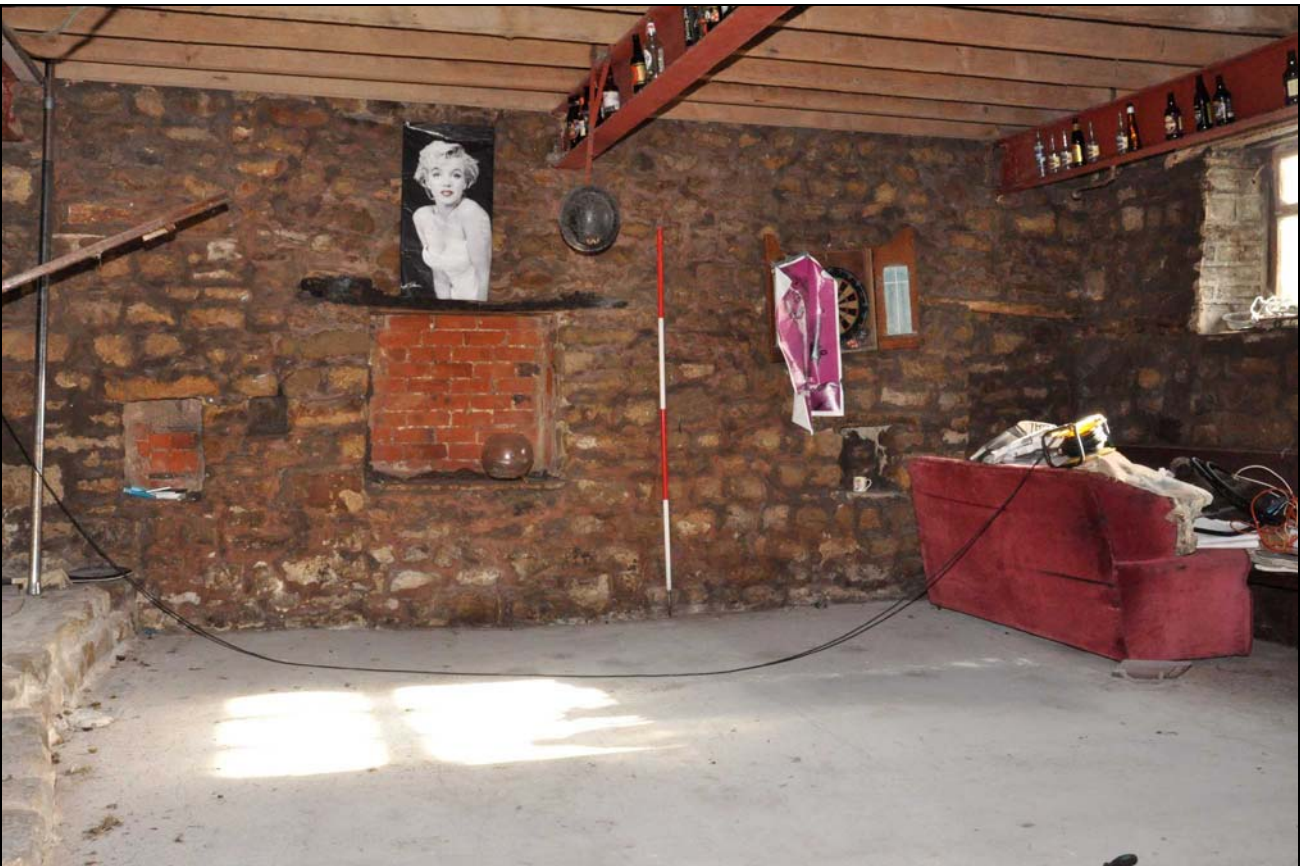
Photo 18: Interior of barn, ground floor, east wall, south end
