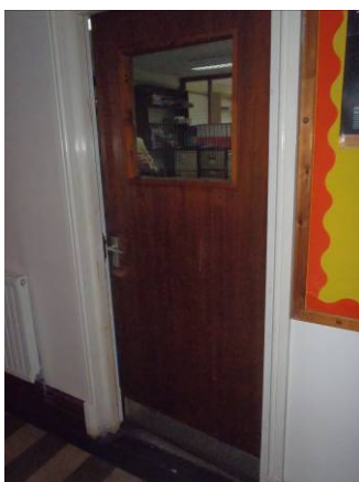
Door 6 Prep Room
