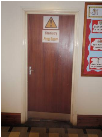
Door 11 Prep Room
