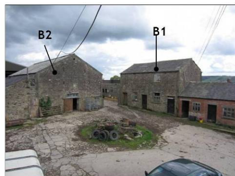
Photo C: Building 1 (north elevation) and Building 2 (west elevation)
