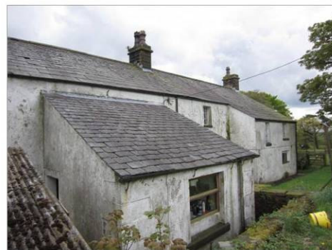
Photo A: Existing farmhouse (north elevation)
