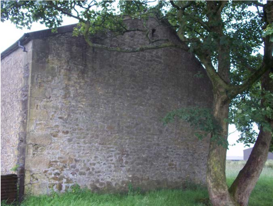
Right Hand Elevation Showing proximity of tree
